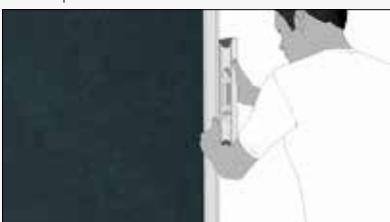
**4- For laying the sheet, we recommend you use masking tape, which will have to be stuck to the sheet's edge. This way we will prevent the adhesive to get in the surface when installed, and the excess of adhesive will be easily removable**
