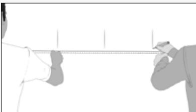
**3- Next, knowing the sheet format, we shall mark the width and height measurements shall on the wall, in order to assist with its installation later.**
