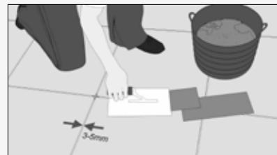
**Filling joints: the installation of tiles without joints should be avoided at all costs. The joint width depends on the tile size. (Minimum values of 3-5 mm.). L'Antic Colonial recommends COLORSTUK 0-4 + cl-Stuk from Butech.**
