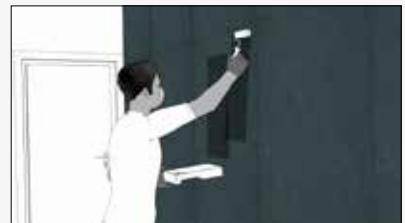
**8- The material is supplied protected, so there is no need to apply any water repellent after installation. In case you wish to apply a new protection layer, we recommend the use of a neutral protector like FILA FOB. Once the protective fluid applied, take out the excess with a cloth or tissue so that the application is even.**
