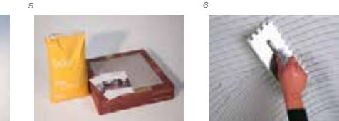
5 Choose the type of adhesive depending on the conditions and tiles used. The choice of tile and adhesive are critical to the subsequent performance of the entire work. Factors to take into account are: the type of ceramic material, tile format, substrate and end use (any traffic it will be subjected to, safety requirements in respect of falls...). PORCELANOSA catalogues contain recommendations in respect of use and slip resistance, as well as the butech adhesive recommended for each design.
